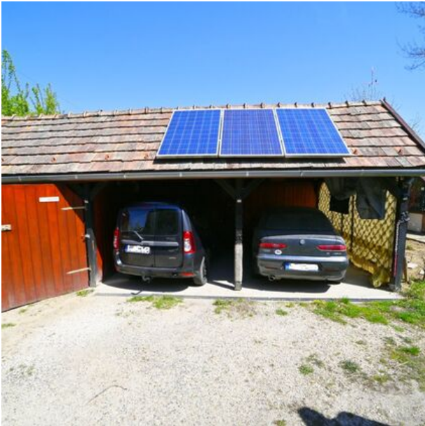
Double garage & shed
