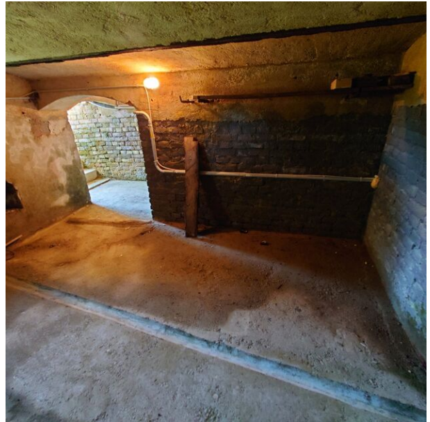
Partial basement under the main house
