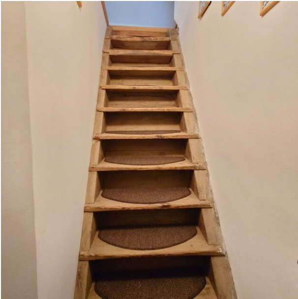
steps to the attic
